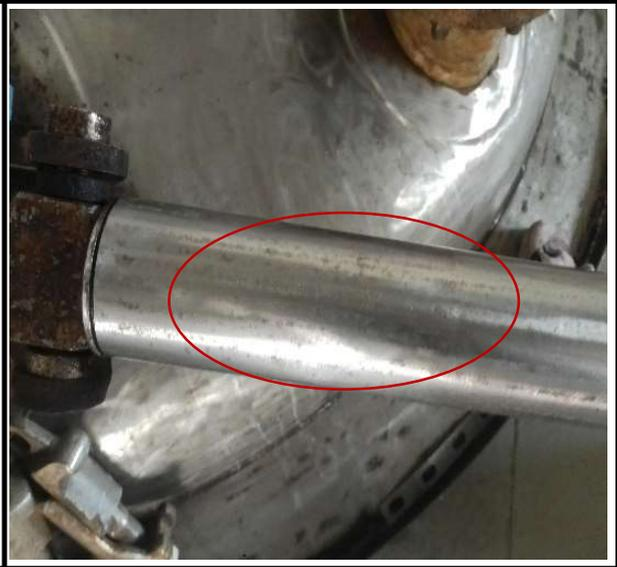
A close-up photograph of the same horizontal stainless steel pipe after cleaning. The surface is smooth, bright, and free of corrosion. A red oval highlights the same section of the pipe.                                          |
