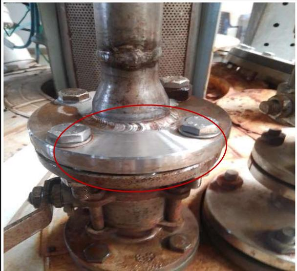
A photograph of the same utility skid pipe flange after cleaning. The metal surface is now bright and shiny, with the corrosion removed. A red circle highlights the same central area, showing the significant improvement in cleanliness. |
